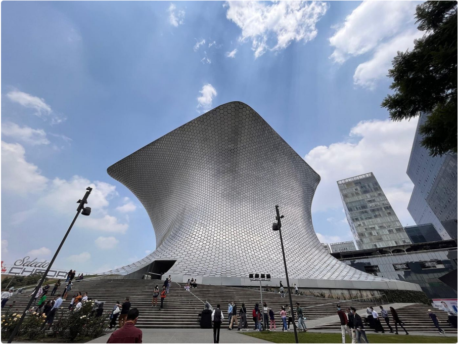
Figure 11.1. Soumaya Museum, Mexico City (2011). Its facade of hexagonal aluminium panels required model-based fabrication coordination.
