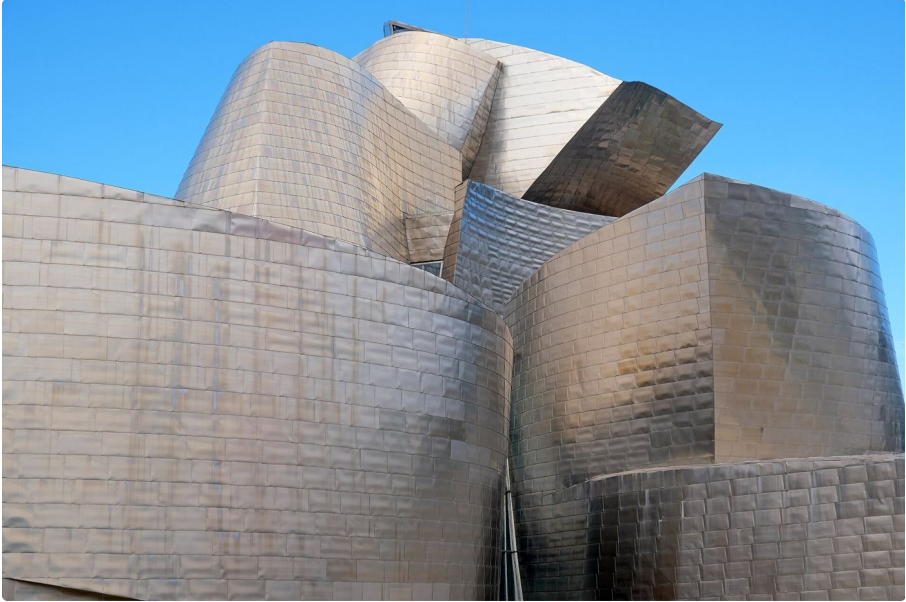
Figure 6.3. The Guggenheim Museum Bilbao (1997). Its titanium curves were engineered and fabricated from a digital model rather than from conventional drawings alone.
